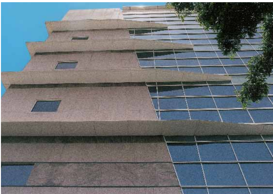
CONSTRUCTION BOOM: The real estate sector has emerged as the flavour of the season
